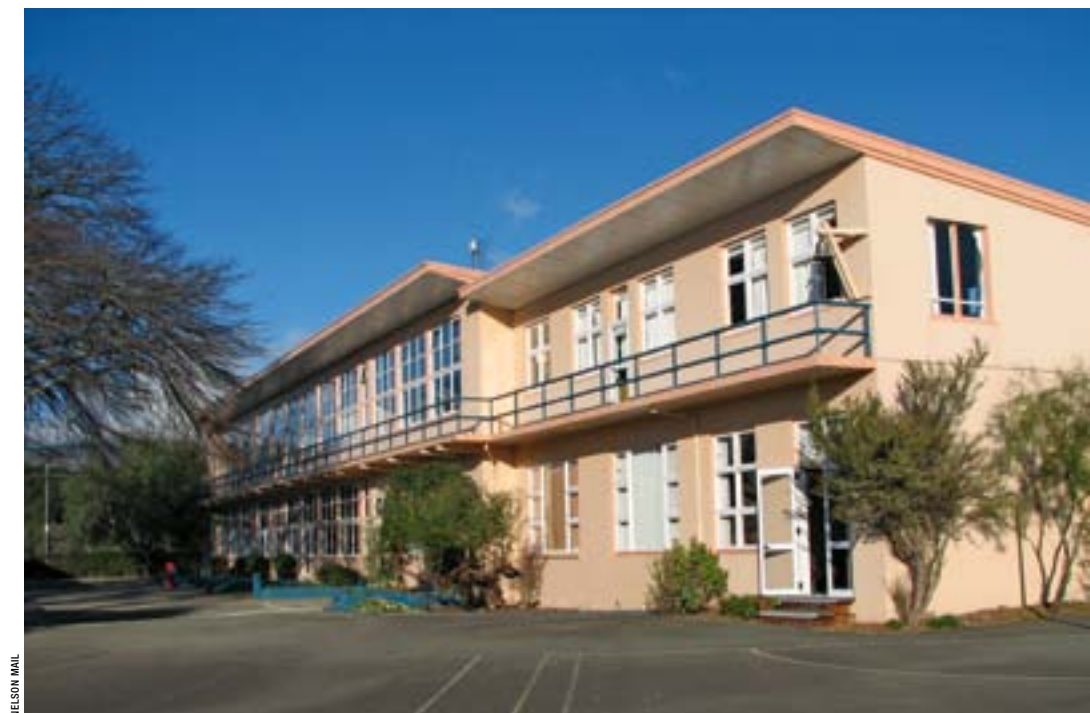
The only "quake-prone" school building in the country to be declared unsafe is the main classroom block at Golden Bay High, in Takaka, vacated in July.
